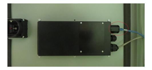
Connect one end of an Ethernet patch cable to the Ethernet port on the HMI, and the other end either to a switch connected to your network (see section 5.9 on how to set up the Ethernet port to communicate on your network).
